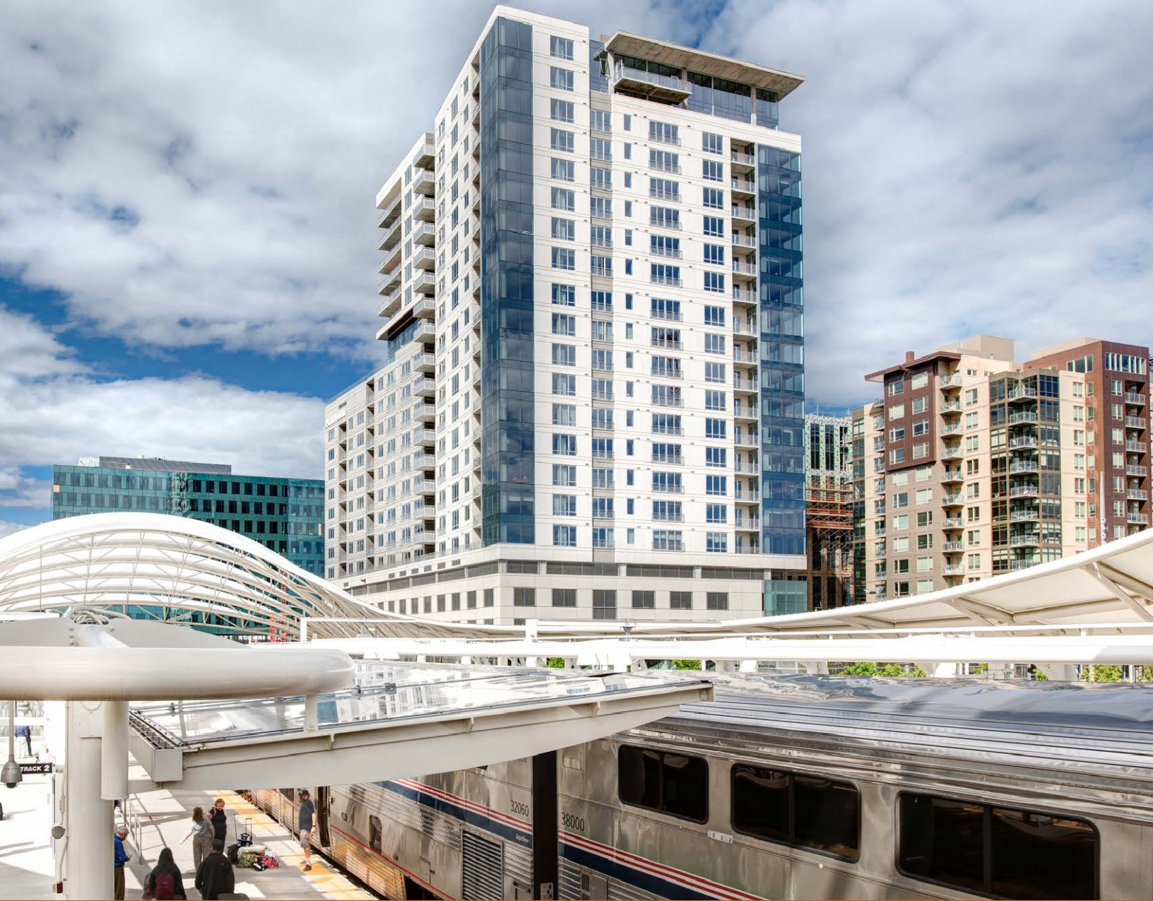
Fund VI | Griffis Platform Union Station | 287 Units | Denver, CO
